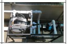
**Stage #3 – Automatic Water Treatment Chemical Dosing System** Supply and fit an ACDS to chemically treat the cooling water in
